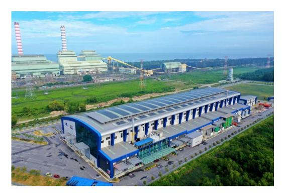
GSPARX had completed installing solar panels on the rooftop of Malaysia Transformer Manufacturing (MTM)'s premises in Kapar and Ulu Klang, Selangor in May 2022. The solar PV installations, under a 21-year Supply Agreement for Renewable Energy (SARE) agreement, are capable of delivering 945 kWp and 532 kWp of solar capacity at Kapar and Ulu Klang locations respectively.
